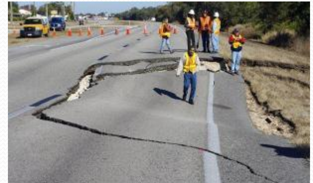
Damage caused by a sinkhole on Highway 27 near Interstate 4 connecting Tampa and Orlando, which resulting in the closure of three of four lanes on January 13, 2010. (Source: Picture by WMG-TV Jacksonville, 2010)
