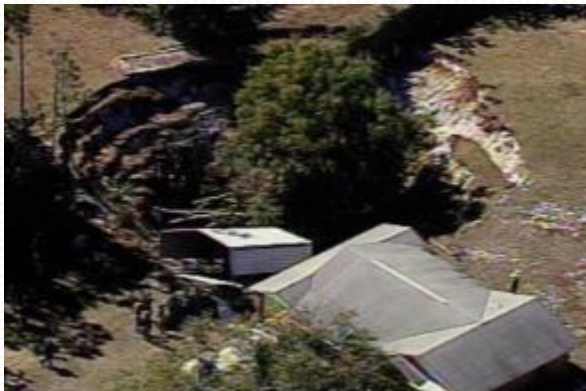
Picture illustrating how a 30 yard wide 40-50 foot deep sinkhole destroyed property in Plant City, FL (Source: Picture by Jay Nolan 2010)
