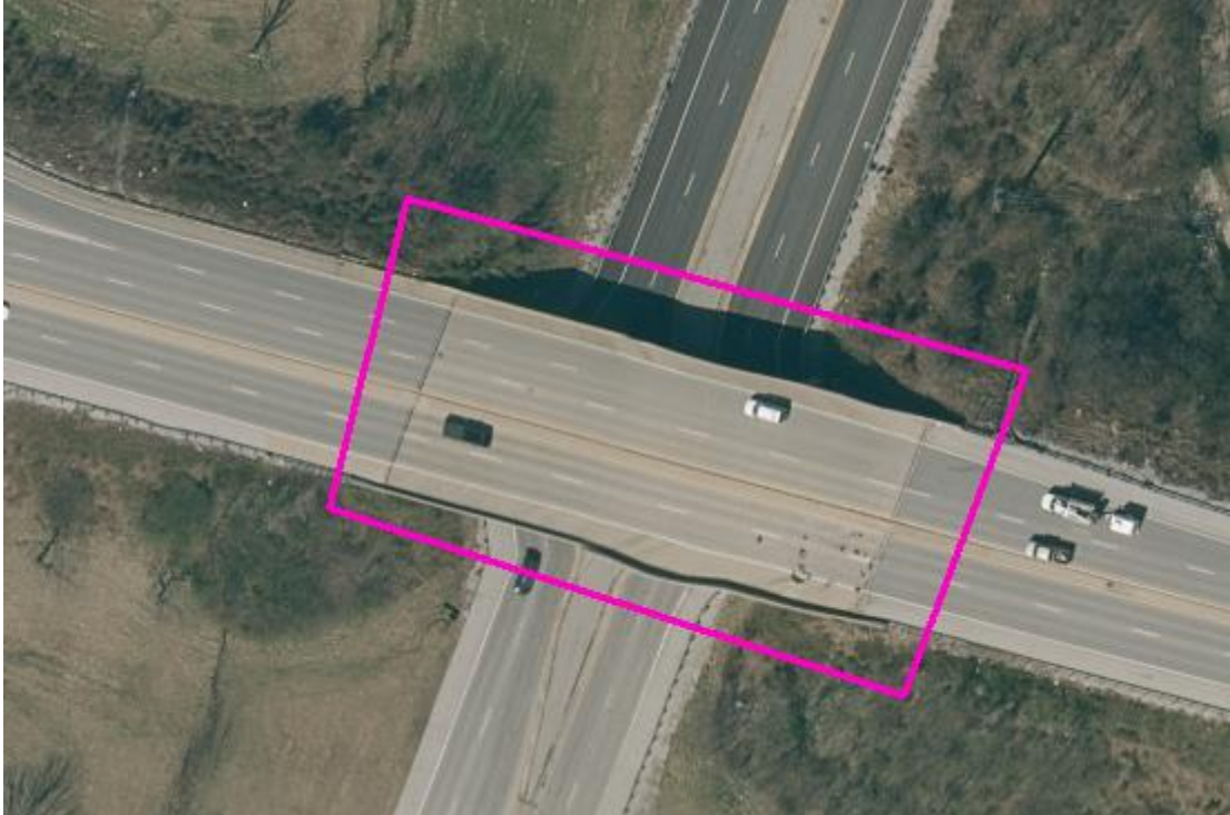
Appendix 3. Example of Bridge Warping in Orthoimagery
