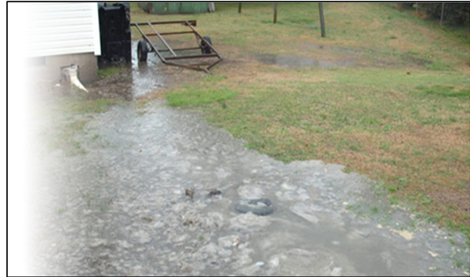
Figure 1. Example of Sanitary Sewer Overflow (SSO).
