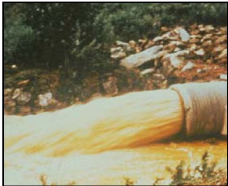
Figure 3: Introduction (Watersheds and Development) - Stormwater Outlet. Legacy infrastructure increases stormwater volume and velocity. (Schuler 2005)
