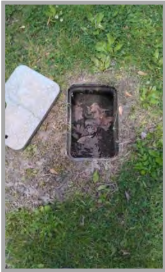
Water hook-up "vault" at campsite
