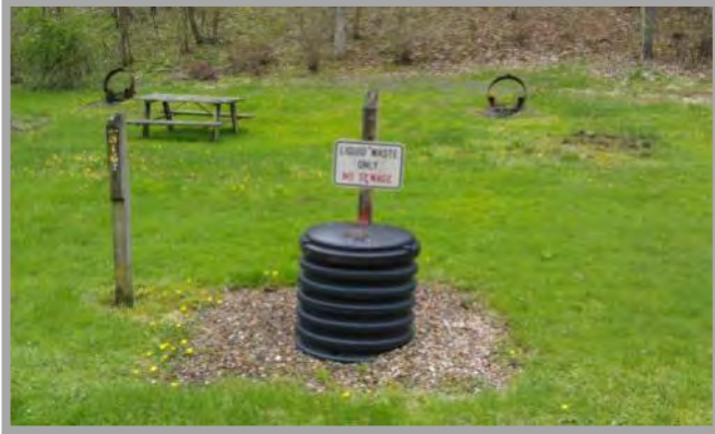
"Gray water" dump station
