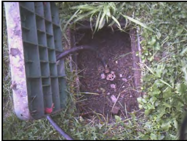
Figure 9: Water service at campsite. Waterline is run into plastic vault and terminated with residential style valve to connect garden hose to a camper. Photograph by Bodo & Associates, Inc.
