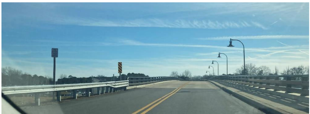
Bridge over Neal Sound to Cobb Island
