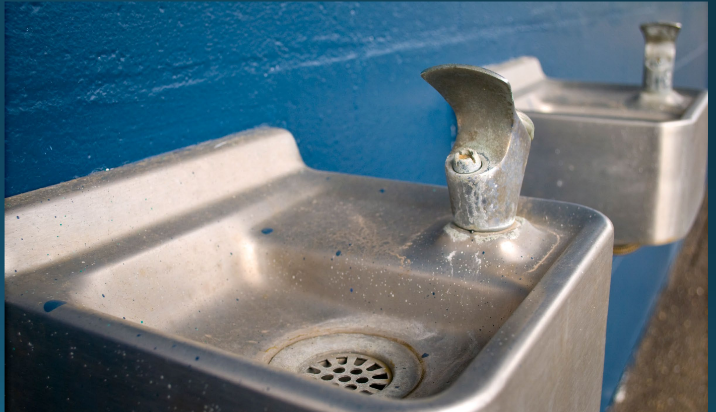
Example of school water fountain that could contain lead solder ( https://nylcv.org/wp-content/uploads/4597707006_973db8e73a_o.jpg )
