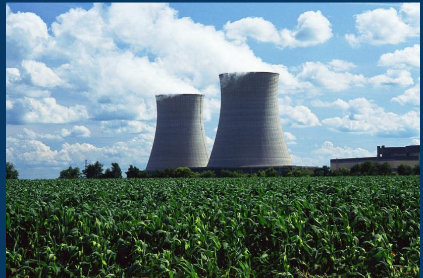
Byron Nuclear Generating Station
