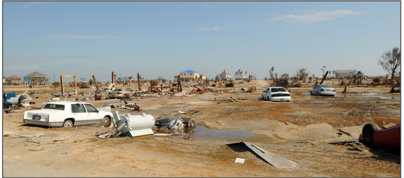
Hurricane Ike damage, Bolivar Peninsula, TX (Credit: Jocelyn Augustino, FEMA)
