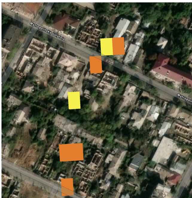
Fig. 10 Instance of building damage not detected in Mariupol, showing limitations in the assessment process and using 20 meter resolution
