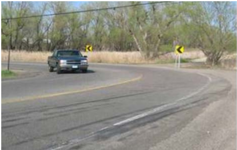
Paving and / or Widening Shoulders
