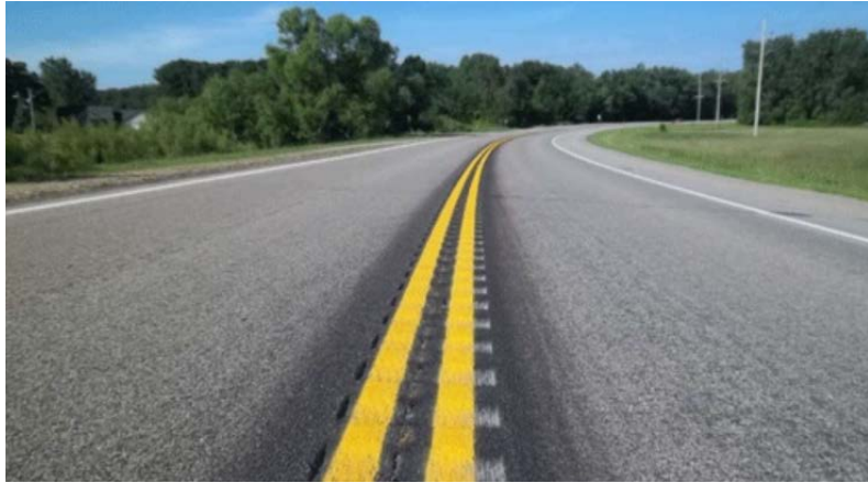
Centerline Rumble Strips
