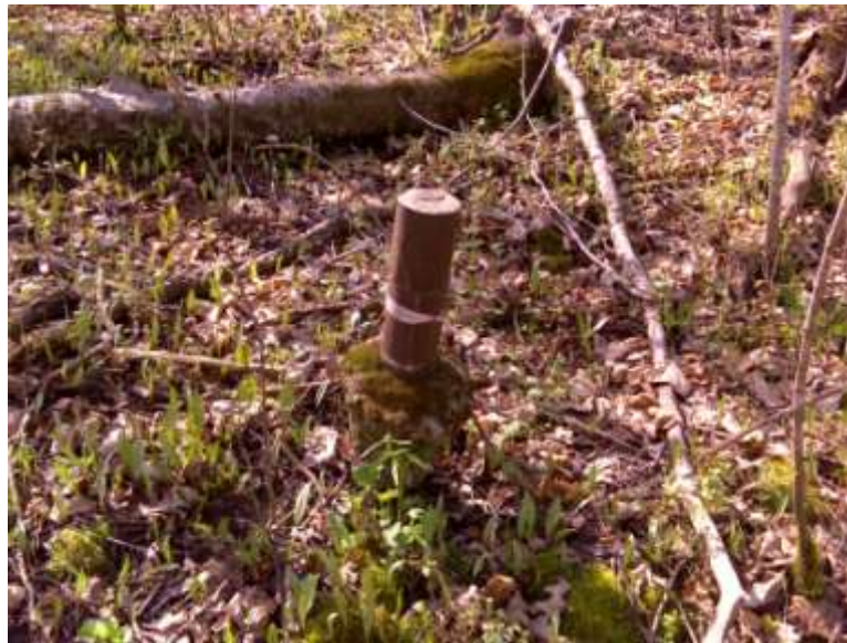
Monument N-2-S. Located 5/6/11. Also referred to in the survey notes as N-2-S. Notice the height of original ground based on concrete level. Unsure if the monument is pushing up or the land is eroding down around the monument. It is near a private campground and there is potential of disturbance based on the fate of other monuments near similar campgrounds. Photo by author.
