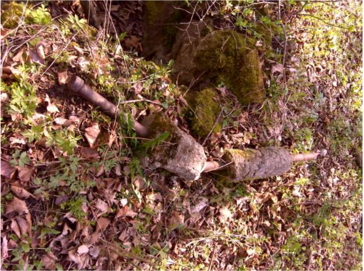
Monument N2-N has been destroyed and was lying on the ground. Located 5/6/11. You can also see remnants of the stone foundation of the house that was in the area. Its position assumed based on location of monument N-2-S, length of x-section range and azimuth from original survey. Photo by author.
