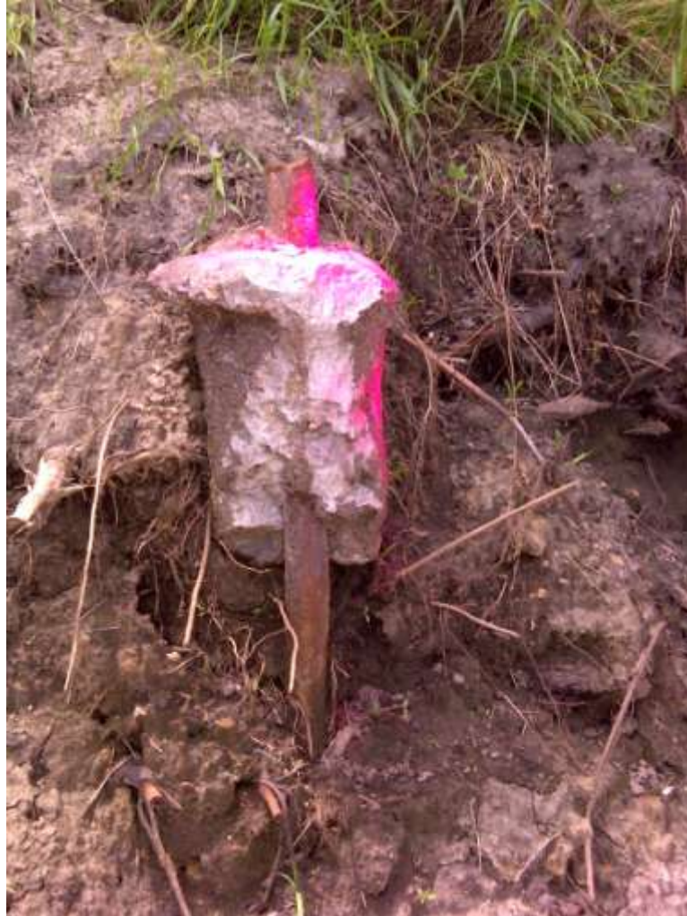
Monument NF-0B. Neither monument could be located involving a number of visits. Located 6/27/11. NF-OB-W was discovered after a visit at the site of a recent excavation. Approximately 3 feet of the monument was exposed and partially damaged. Absolute elevation and latitude-longitude is suspect due to the damage. Photo by author.
