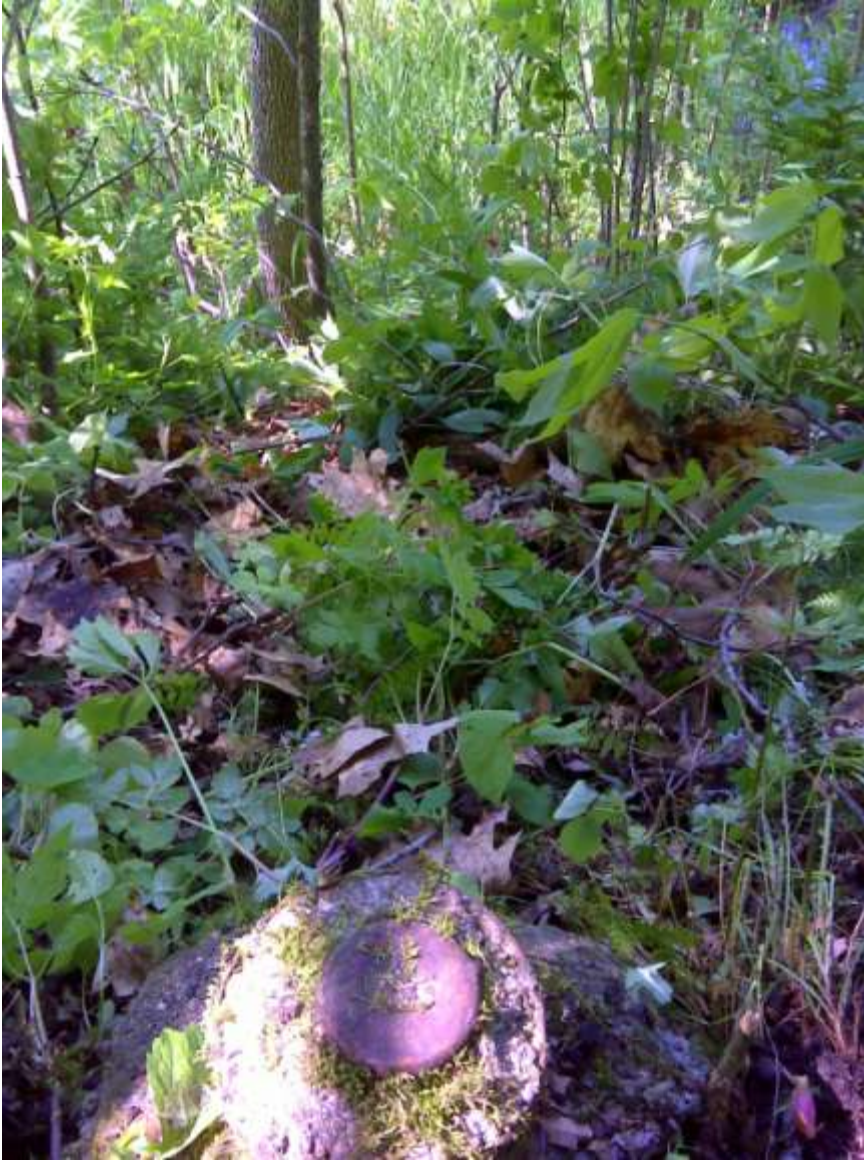
Monument 2-S. Located 5/26/11 Beginning point 0+00 of Range 2 Looking in approximate direction (NNW) of X-section. Even by the end of May the heavy vegetation would make any type of survey during the summer months almost impossible. Photo by author
