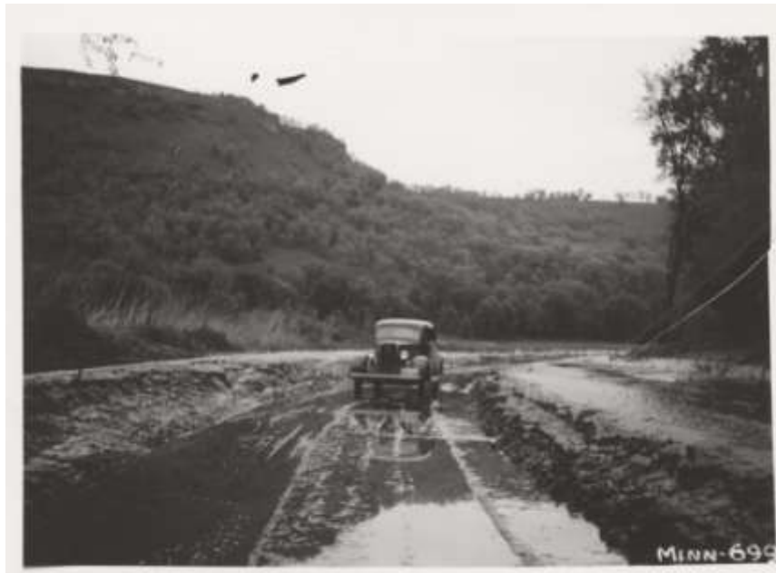
Figure 7 Road Damage due to flooding and sedimentation in the Whitewater Valley. Photo courtesy of USDA Soil Conservation Service.
