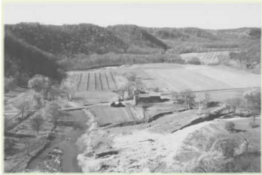
Fairwater Crossing cir. 1940. This is the location of Range NF-2. The photo was taken 1 year after the establishment of the range. Monument NF-2-N was located very near the center of the photo. According to the original notes it was close to the foundation of the house located on the back side of the road. Monument NF-2-S is located out of the photo to the left. Photo courtesy of the Whitewater River Watershed Project.
